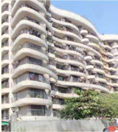
Aditya Vardhan- Andheri East
