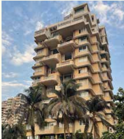
Ritu Apartments - Bandra West
